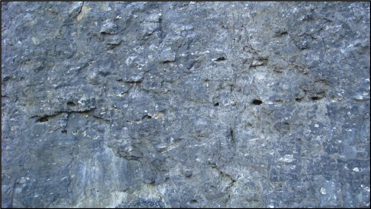
Plate 7-9: Close-up of Plate 7-12 showing weathered 'vuggy' cavities, unconnected
