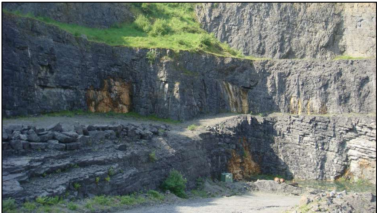
Plate 7-20: Groundwater inflows at southwest corner of quarry (epikarst higher up face)
