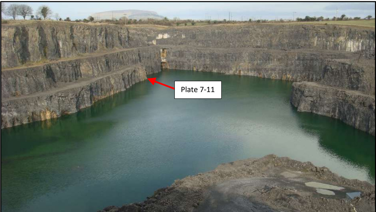
Plate 7-10: Location of only deep weathered zone noted in quarry
