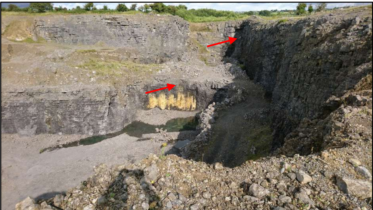
Plate 7-18: Groundwater inflows from epikarst at northeast corner of quarry
