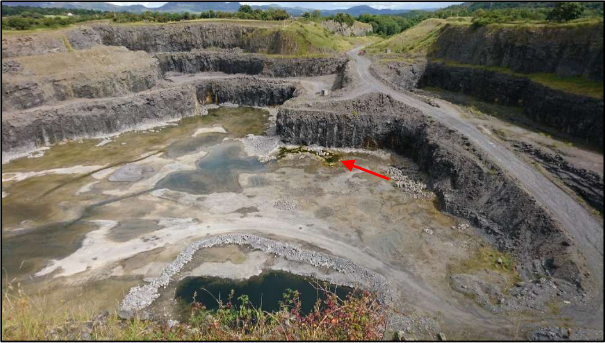
Plate 7-21: Groundwater inflow on quarry floor, elongate along quarry wall (rising of groundwater flow along bedding planes)
