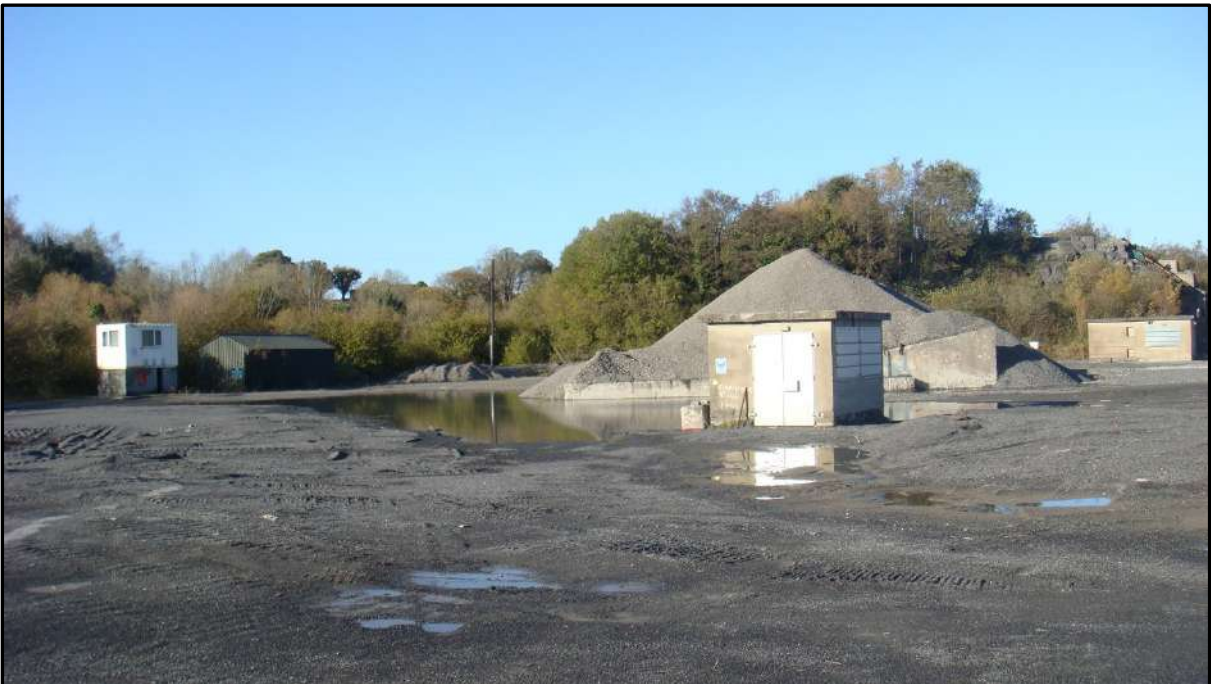
Plate 7-4: Eastern part of application site (note ponding due to heavy rainfall)
